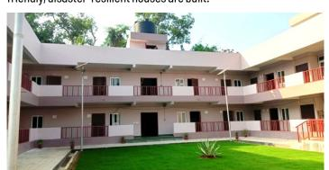
In the newly-inaugurated project, 40 (G+1) houses have been constructed using 'Structural Stay In Place Steel Formwork System' technology. The building is equipped with all basic and modern facilities, including a medical room, office, caretaker room, dining room, kitchen and activity room.
